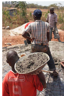
Construction of a Rainwater Tank/ Kagera Tanzania
