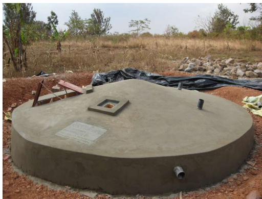
Rainwater Tank/ Kagera Tanzania
